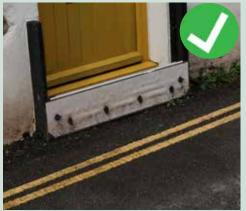
**Figure 68:** - Active control method, flood gates can be quickly setup.
