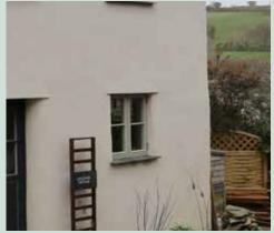
Figure 61: - Wall construction - average thermal transmittance 0.13 W/m<sup>2</sup>K (EPC Very Good)
