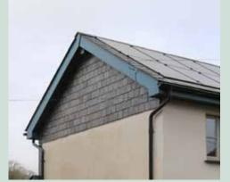
**Figure 62:** - Roof construction - average thermal transmittance 0.15 W/m<sup>2</sup>K (EPC Good)
