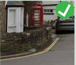
**Figure 67:** - Dwarf wall boundaries can provide subtle water control in combination with flood gates
