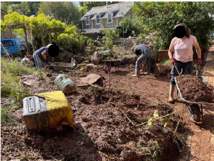
St Clement's Terrace clean up
