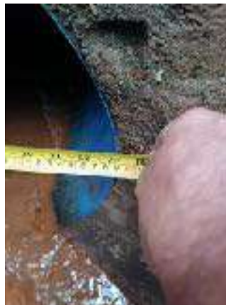
St Clement's culvert 590 mm
