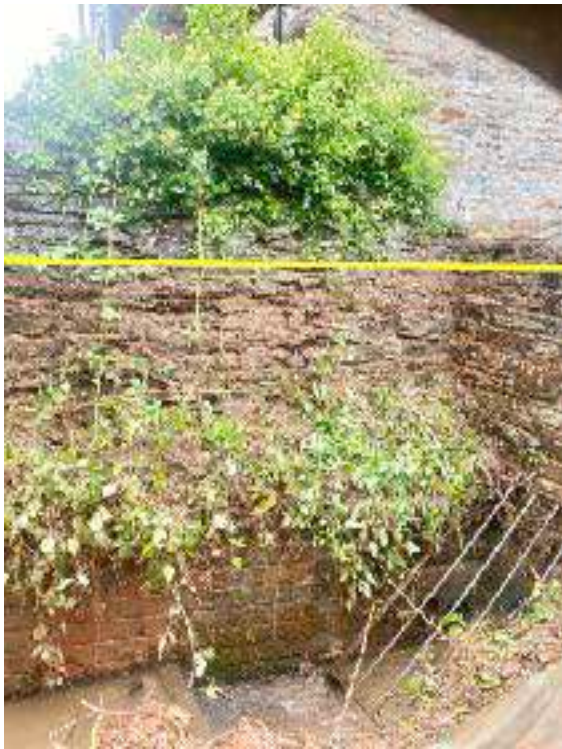
Inclined grating over the culvert
