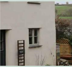
**Figure 62:** - Wall construction - average thermal transmittance 0.13 W/m<sup>2</sup>K (EPC Very Good)
