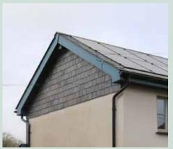
**Figure 63:** - Roof construction - average thermal transmittance 0.15 W/m<sup>2</sup>K (EPC Good)
