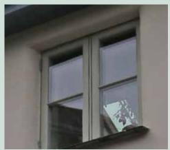
**Figure 61:** - High performance glazing. windows and doors are all triple glazed
