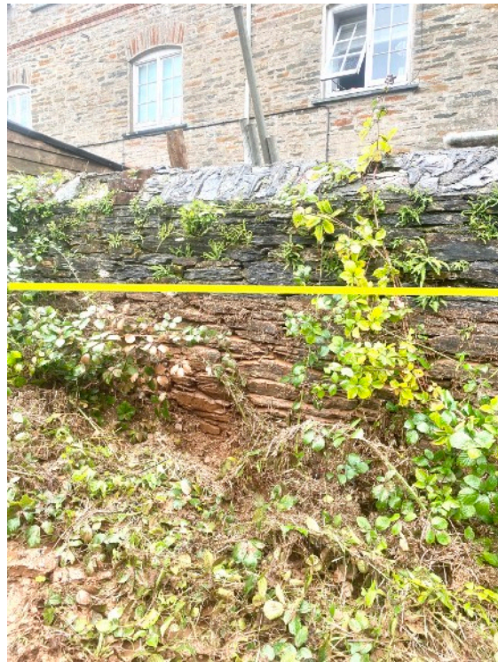
St Clement's rear wall
