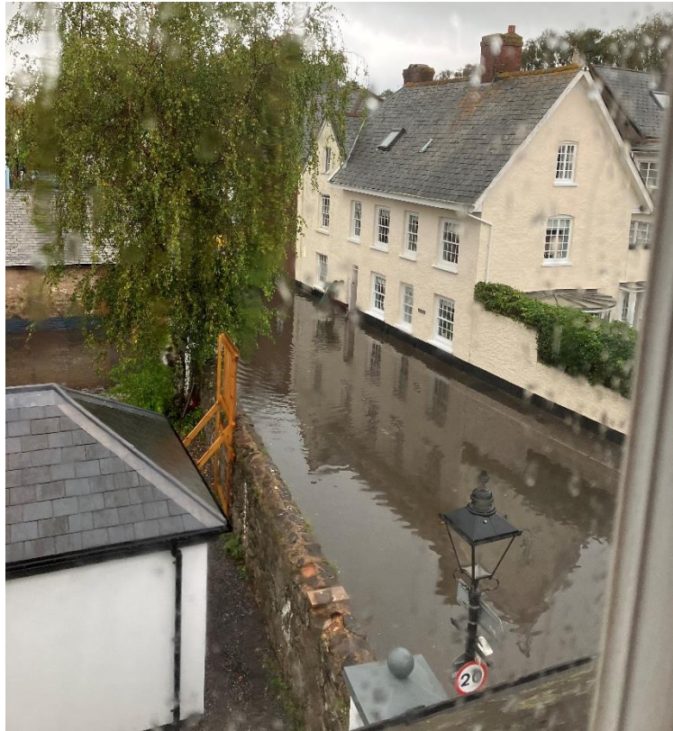
Figure 5.4. surface water on Ferry Road, Topsham 17 th September 2023. Credit: Topsham resident
