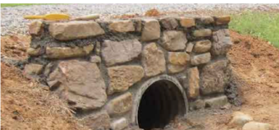
Examples of bank retention around a culvert
