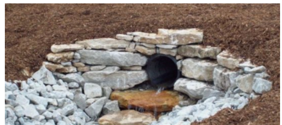
Examples of bank retention around a culvert
